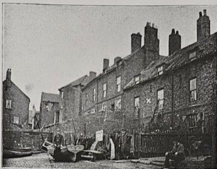
Fig. 3. John Walker's Private House at Stockton at the present day. (House marked by a "x.")
